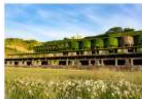
KITAZAWA FLOTATION PLANT
