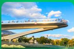
Floating Bridge Moscow
